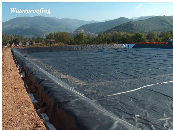
**Figure 20** Impermeable soil cover.
